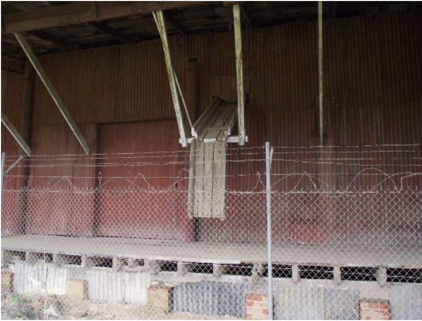
Above: Loading dock, door, and loading chute.
