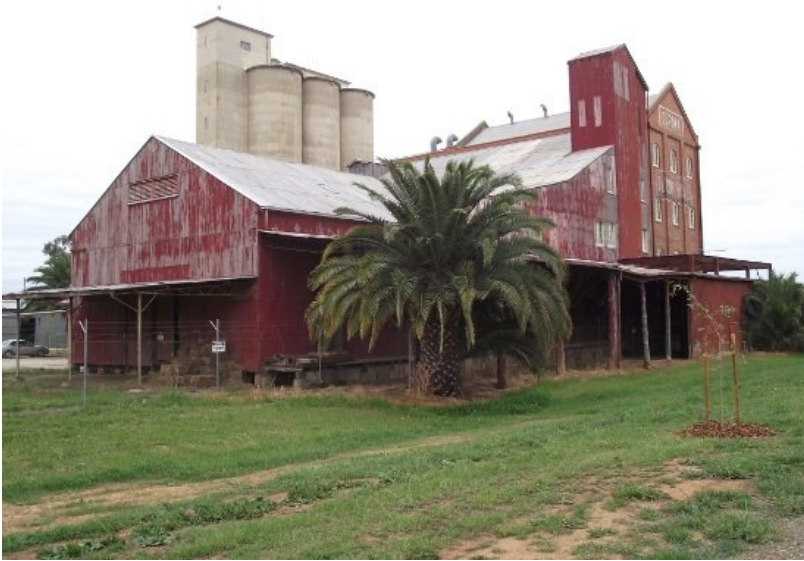
Above: Overall view of railway side of building, showing the loading dock and other features.
