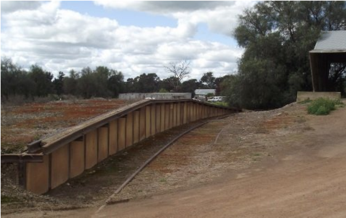
Above: Silo platform
