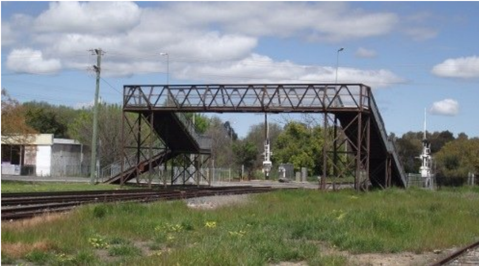
Above: Footbridge, looking south towards Albury
