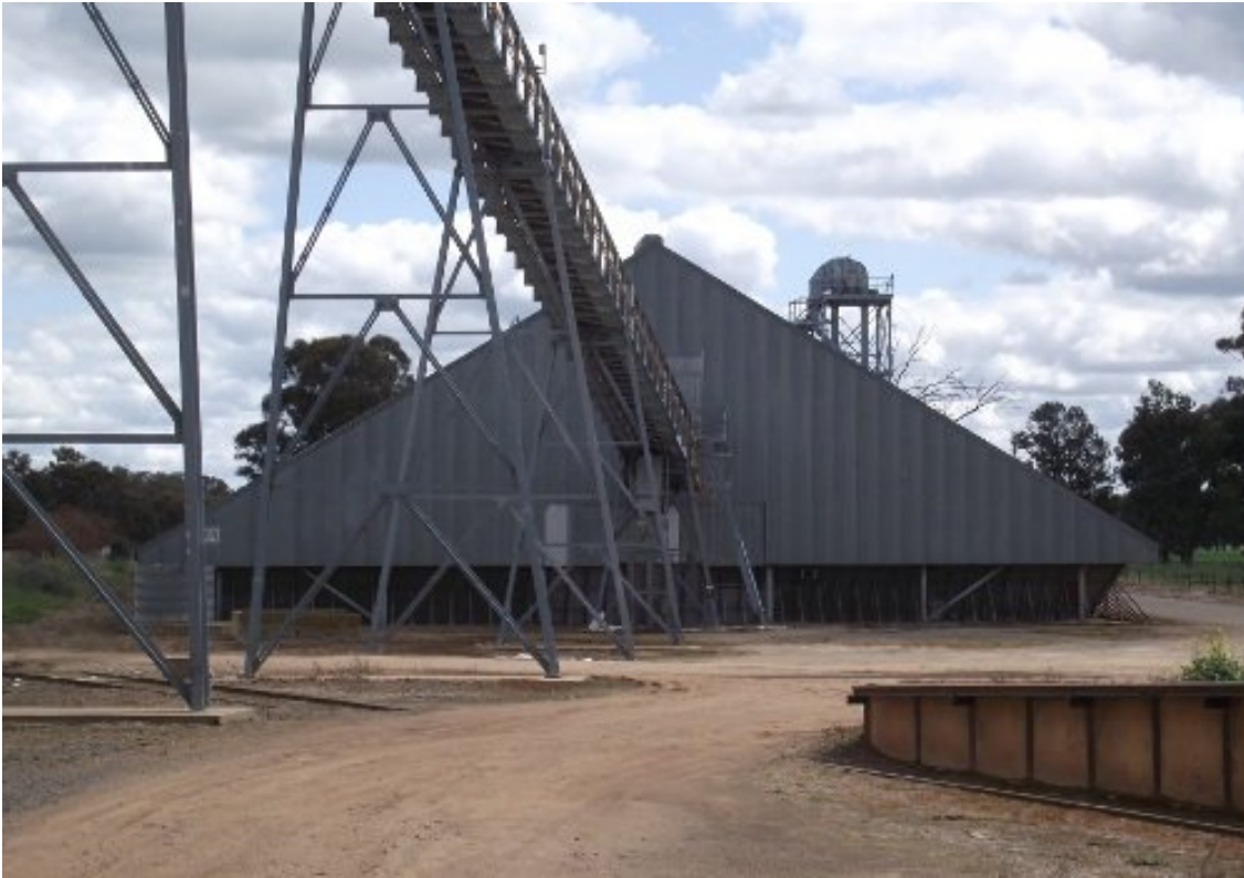
Above: Silo shed
