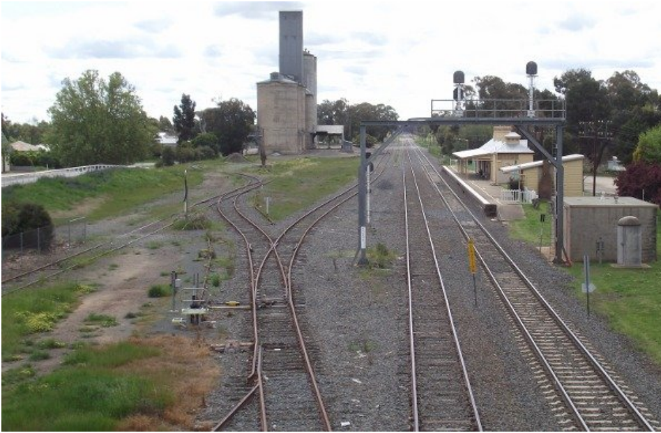
Above: Looking north from footbridge towards Wagga Wagga
