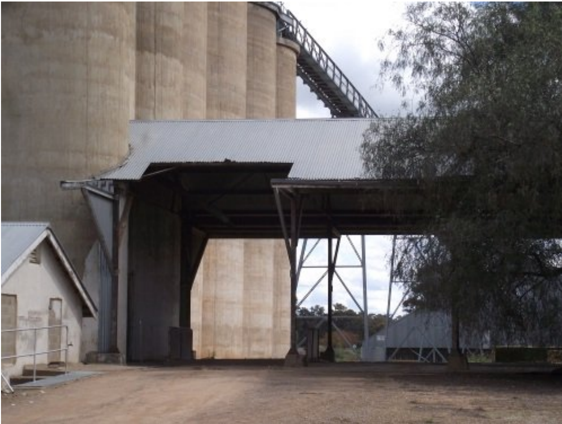
Above: Silo road vehicle unloading shed
