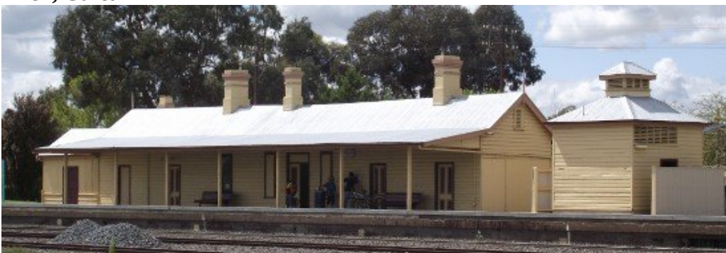
Above: Station building
