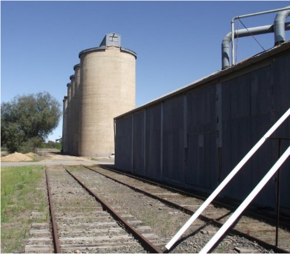
Above: Silos, track and shed
