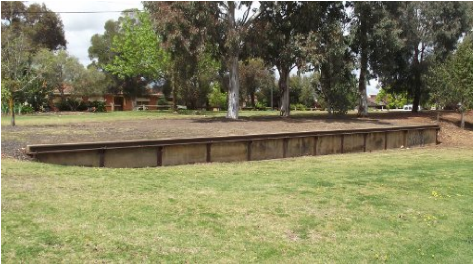
Above: Extra platform at station.
