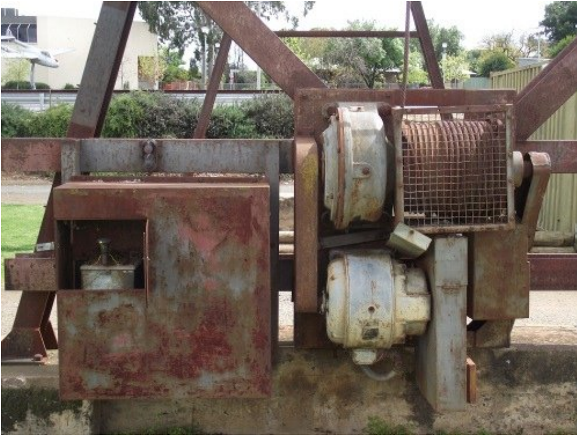
Above: Gantry crane mechanisms
