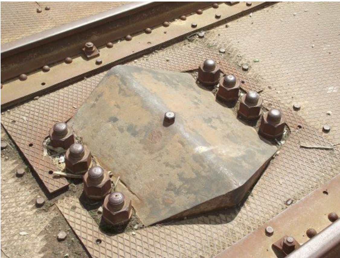
Above: Large bolts for the turntable pivot.
